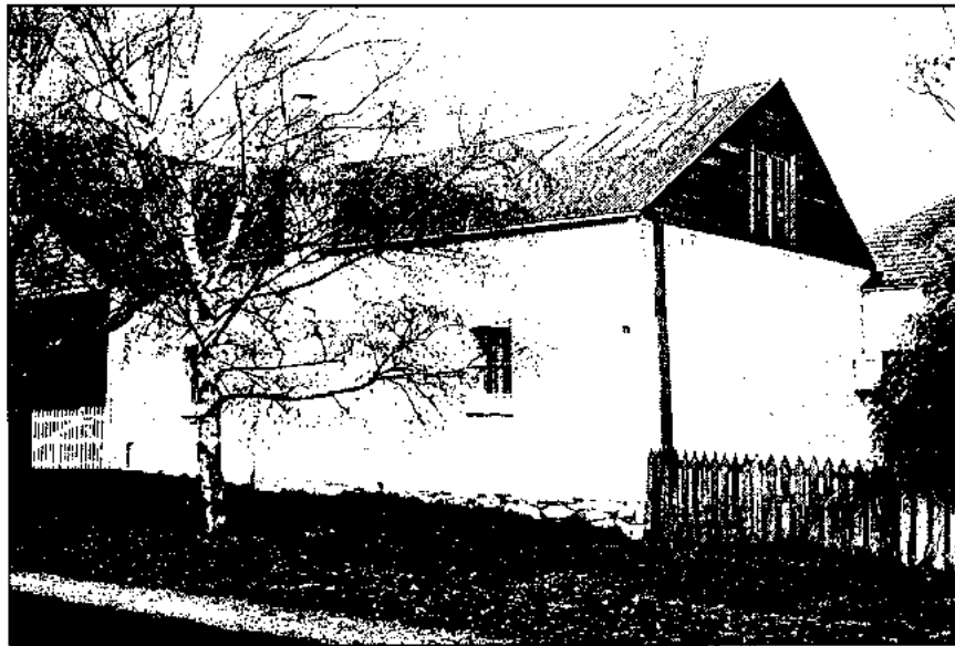
Remains of Westfield Mill, Westbury, 1997. The top storey was removed some years ago.
