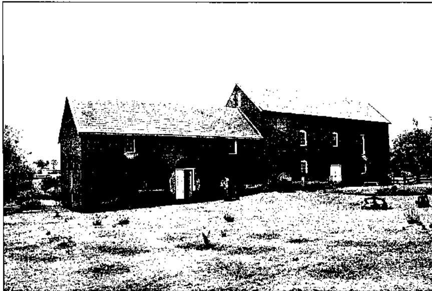
The second Thorpe Mill, Bothwell, 1998, showing the head race coming in from the right.
