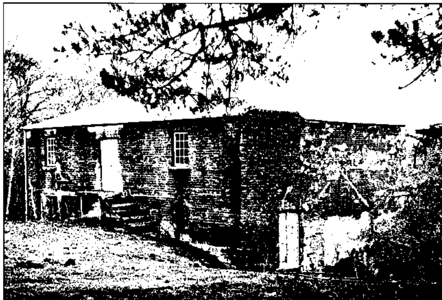
Strathmore Mill, now Lochmaben, near Evandale 1985.
