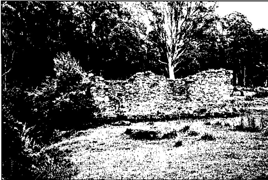
Stone remains of Egmont Mill, Westbury, 1996.
