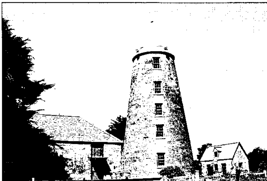
Callington Mill complex, Oatlands, 1997. The wind- mill, with reconstructed cap, is flanked by the steam mill (left) and the miller's cottage (right).
