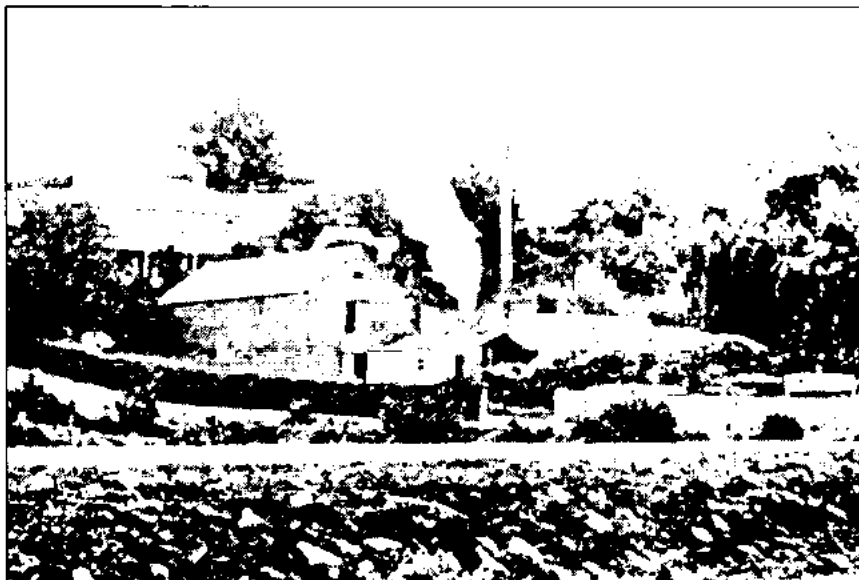
Shorey's/Harvey's mill, Deloraine, c.1900. The engine house and other surrounding buildings have now gone, but the mill building survives in good condition.
