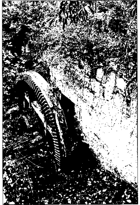
Remains Clarendon Mill, Derwent Valley, 1997, showing pit wheel.
